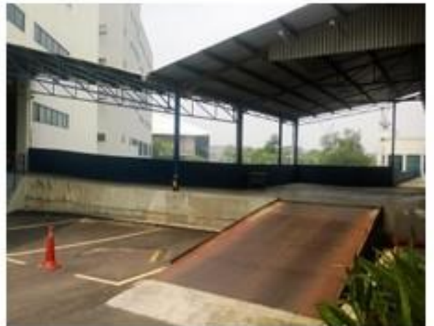
Loading area with 2 loading bays
